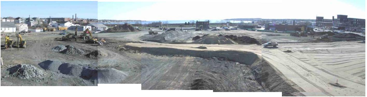
**Description:** Site grade was raised approximately 6 feet to construct a 70,000 SF, 1-story supermarket and loading dock area and an adjoining 7500 SF retail building at the site of a former mill building. Typical interior column loads ranged from 35 to 183 kips with perimeter foundation walls and combination foundation/retaining walls bearing at 2 to 7.2 KLF. Floor loading ranged from 150 to 250 psf.
